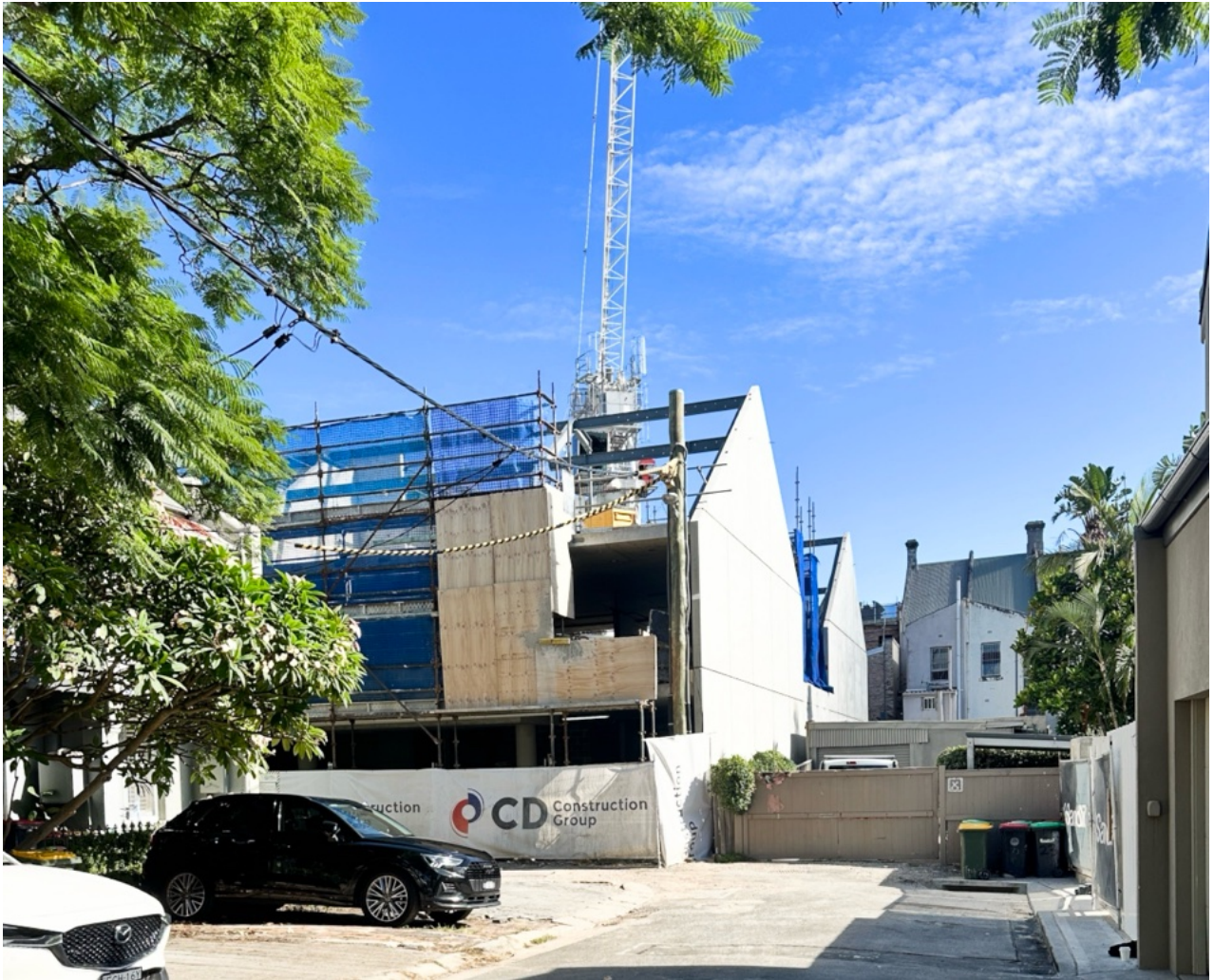
432–440 Oxford from rear. Currently under construction
