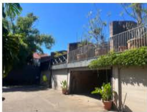
Fig. 41 Access to carparks at 142-148 Oxford Street is from a narrow lane from Gipps Street.
