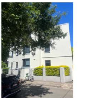
Fig. 46 Shadforth St façade of 160 Oxford Street. Shadforth St and rear façade No. 160 Oxford Street.
