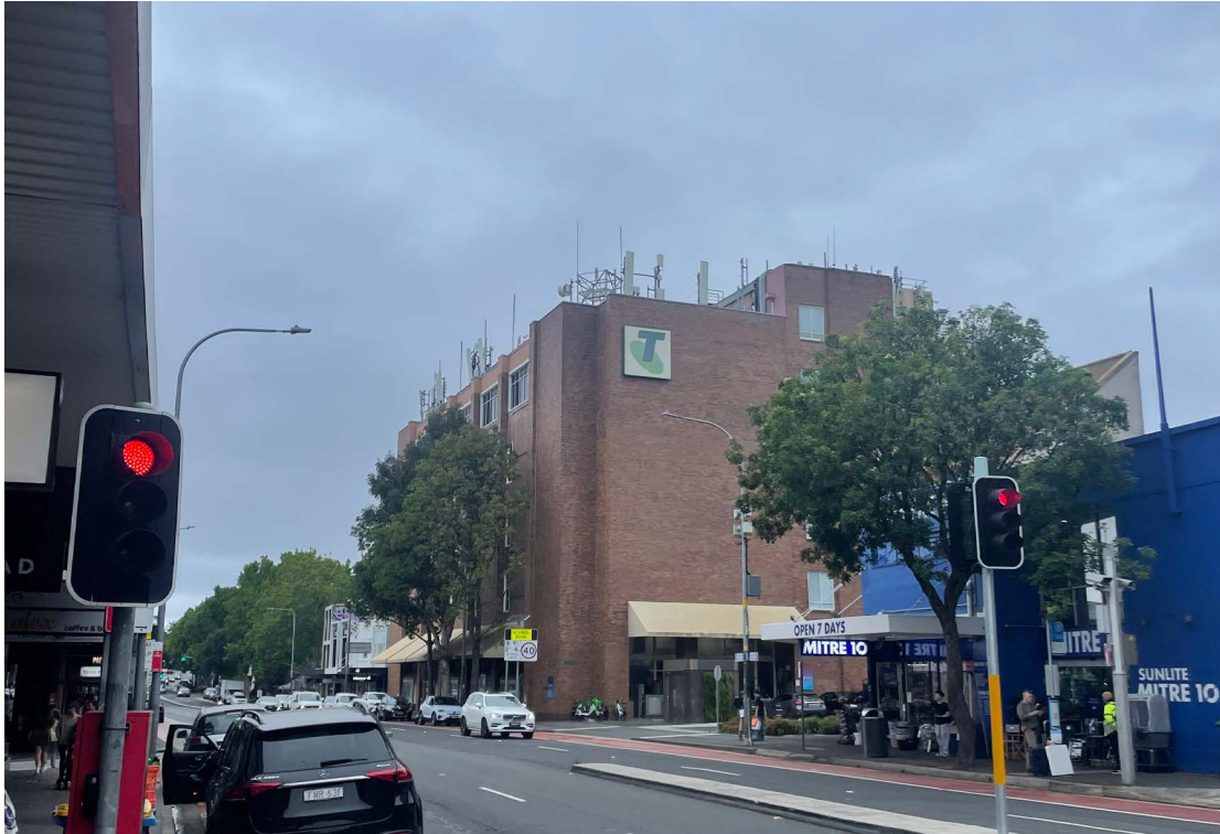
Telstra Building in City of Sydney, 363 Oxford Street.
