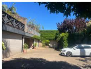
Fig. 43 Access to carparks at 142-148 Oxford Street is from a narrow lane from Gipps Street.
