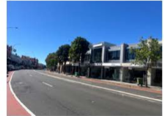
Fig. 28 Contemporary in-fill shops. Southern side of Oxford Street. 2 storeys.
