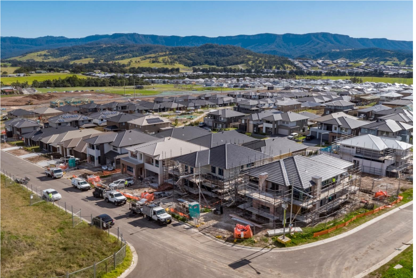
Figure 2: A birds-eye view of a residential subdivision under construction
