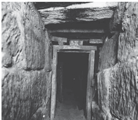
Interior of Busby's Bore – a 3.6 km long tunnel Source: City of Sydney Archives
