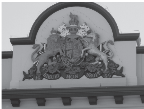
View of the repainted Paddington Post Office
