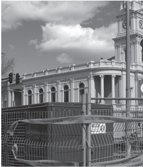
The new Ausgrid substation on Ormond Street.
